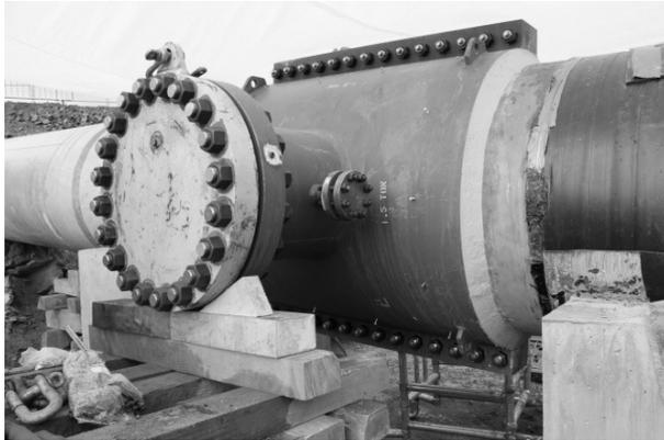
As one of GL Noble Denton's most innovative technologies for pipeline intervention, Grouted Tee introduces an intelligent mechanical method for attaching a new branch connection to an existing flow line.
