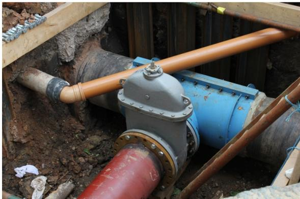
PMC provided guidance on the best repair method on the leaking IP main. The steel main in question was located in the carriageway of a busy A Road in close proximity to a busy junction, businesses and a busy café so it was imperative that the repair was undertaken in a timely, safe and efficient manner.
