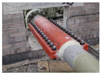
Waring Engineering prides itself on the quality of service and products and has remained GL Noble Dentons prefered supplier for pipeline repair sleeves, Grouted Tees and other bespoke fabrications.
